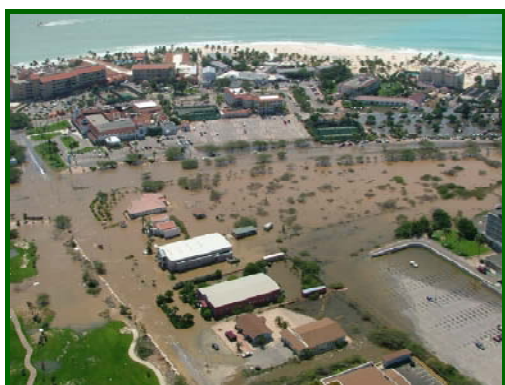
Picture flooded area
